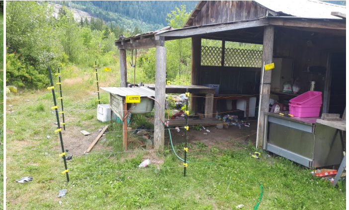
Photo 2: Semi-permanent electric fence around entrance and working area of smoke house (steel stakes and 110v energizer).
