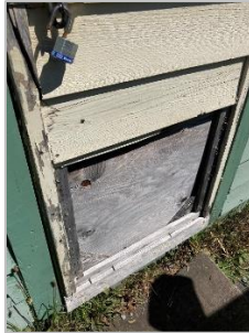
Figure 5. Bear broke through garbage shed door and pulled off hasp and lock.
