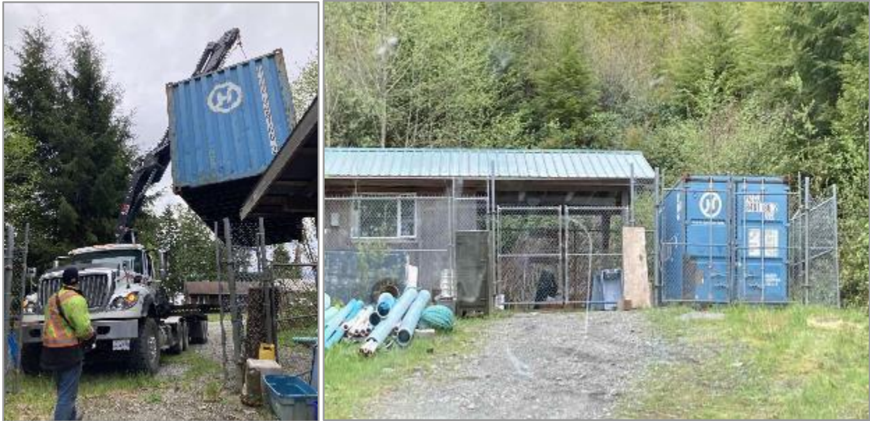
Figure 9. Sea can in Macoah securing the recycling storage facility that had been accessed by a black bear in the past (Left: During the installation, Right: After the installation). Credits: David Johnsen
