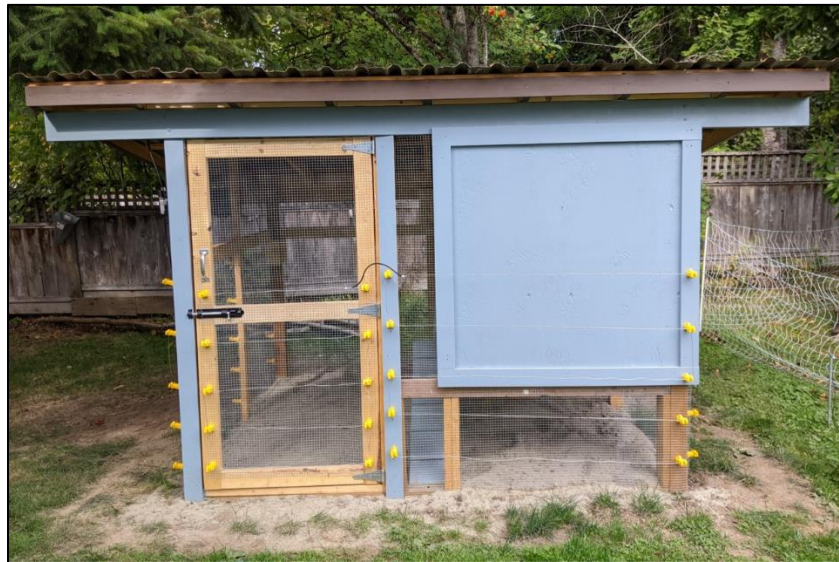
Figure 6. Electric wires outrigged around a chicken coop using materials funded through the WildSafeBC cost-share program.
