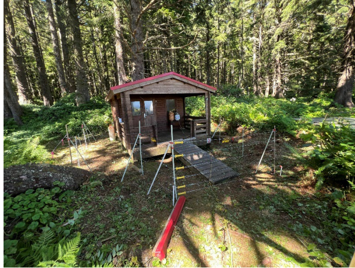
Figure 20. Solar powered electric fencing for a Ditidaht First Nation Guardian patrol cabin.
